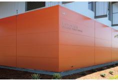
Our flat wall panels are produced with a standard embossed face and offer a perfect solution for designers seeking a high-end architectural look with all the thermal benefits that insulated metal panels offer.
