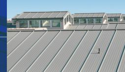
The look of traditional standing seam integrated with the benefits of an insulated metal panel - a great alternative to field assembled roofing components.
